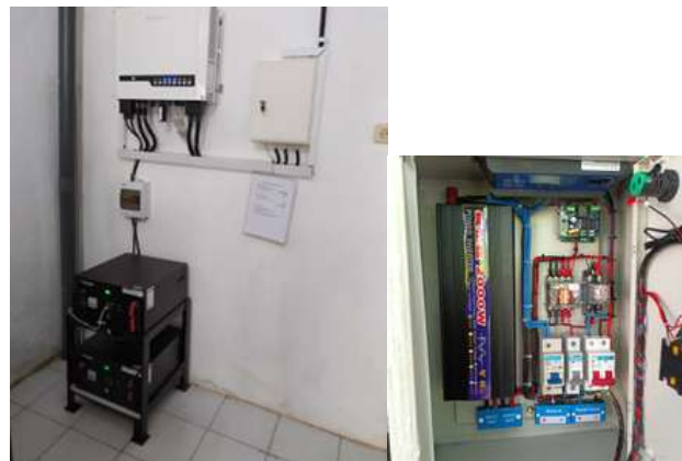
Figure 6. Battery and PV Junction Box
