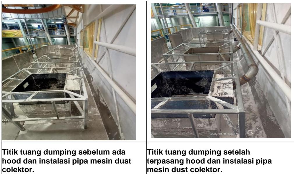
Picture 7 : Repair Process Before and After
